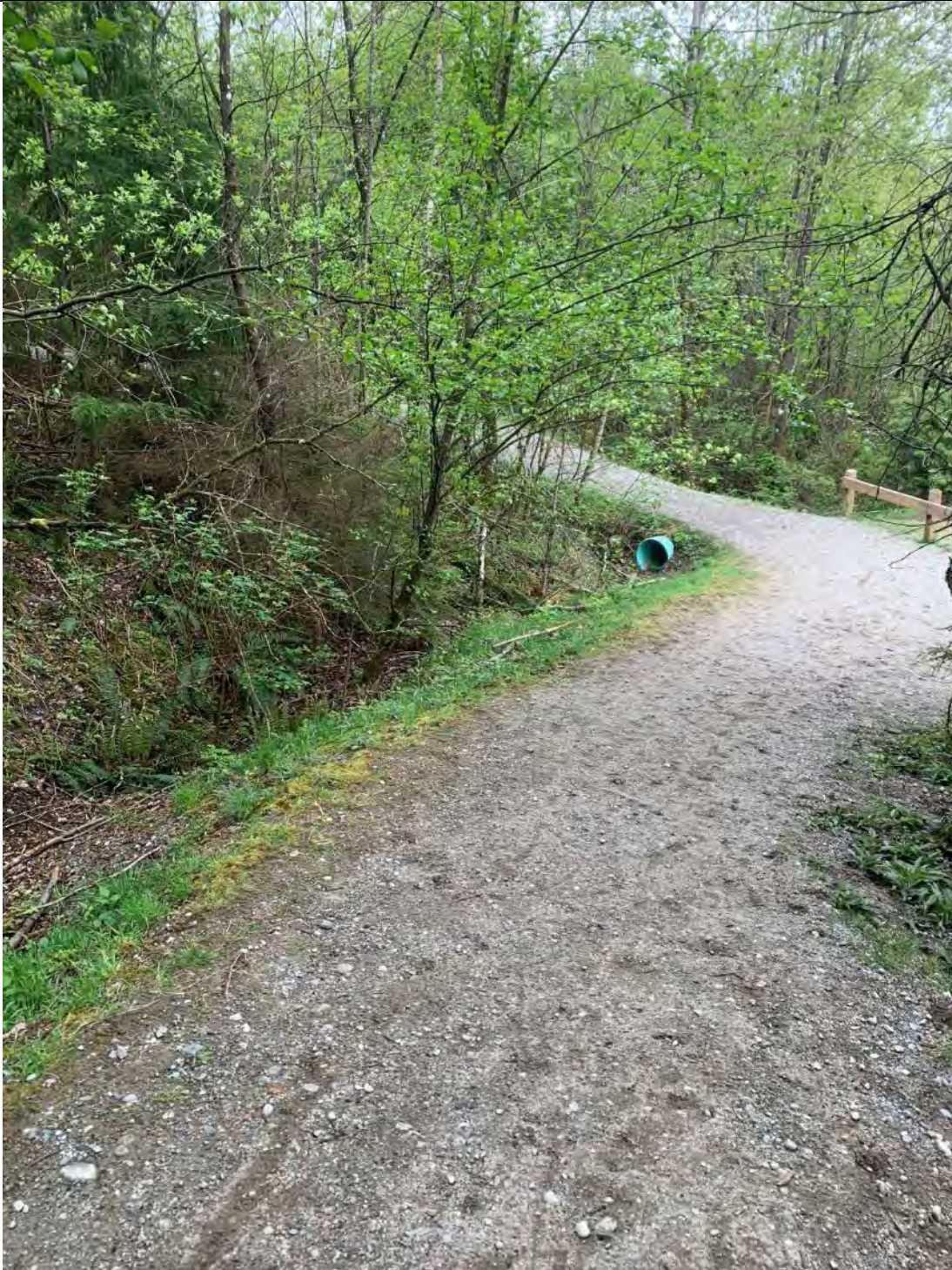
Photo 8: Ditch on the uphill side of the pathway that is above the erosion site. Note the PVC culvert crossing the other trail in an east-west direction.
