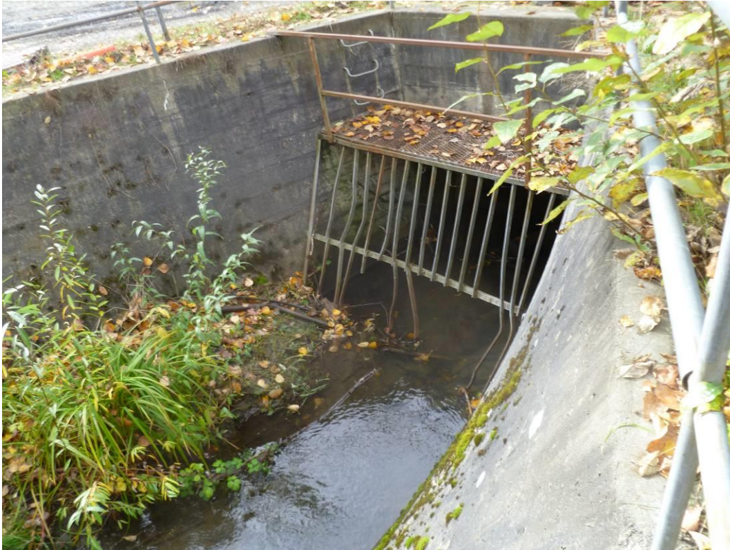
Photograph 25: Suter Brook Creek culvert with grate u/s of railway spur-line.
