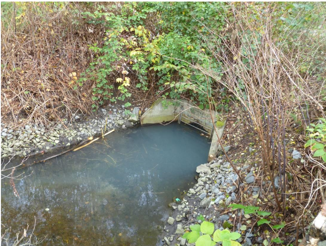
Photograph 20: Suter Brook Creek culvert outfall with oil-water separator, d/s of Murray St.
