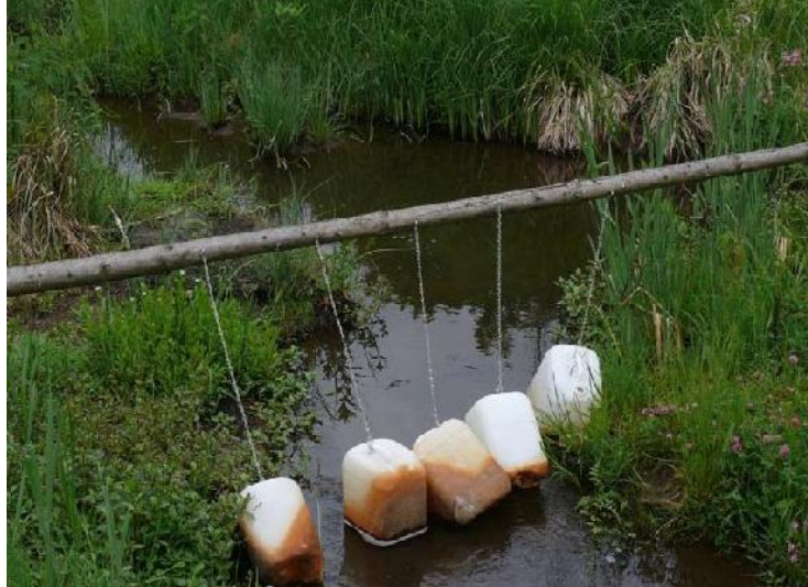
Figure 9. Beaver deterrent installed in notched dam to desired water-level height. Materials include plastic canisters and metal chain (Image: Valachovič 2012)
