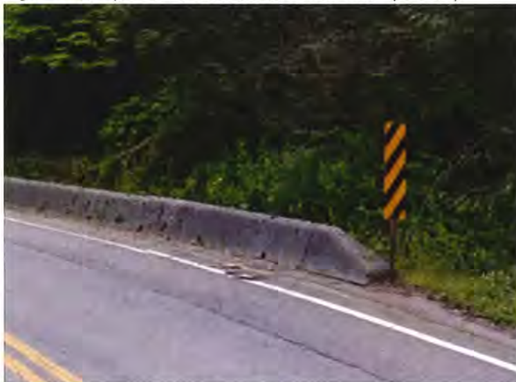
Figure 1: Sample Low Concrete Roadside Barrier (450mm)
