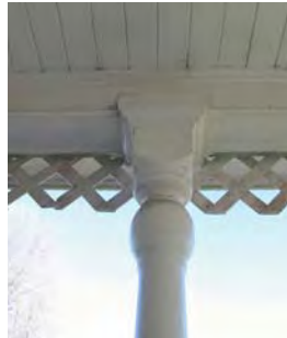
Photos showing top (left) and bottom (right) portion of the typical full lathe turned column and newel post at the front porch. Note the 2x4 addition on above the newel post that is not a character-defining element of Johnston House.
