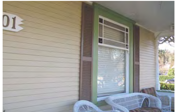
An original double-hung wood-sash window, with multi-pane upper sashes and coloured glass at the western portion of the front porch.
