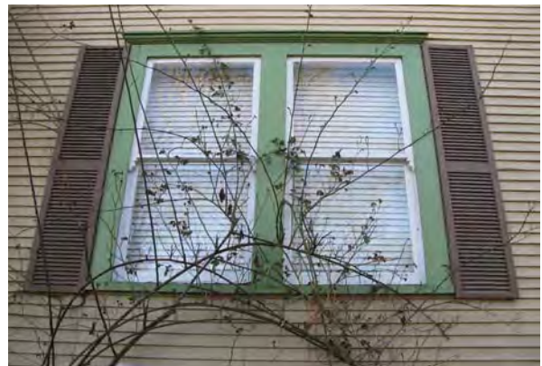
Existing condition of all four original windows at west elevation. Note that all windows on the second floor have similar configuration at west, north, and east elevations. The two ground floor windows at the northwest corner have multi-paned upper sashes and coloured glass.
