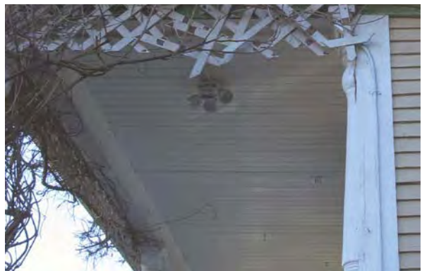
Parallel configuration of closed soffit at the west portion of the front verandah, oriented perpendicularly in relation to the exterior wall.
