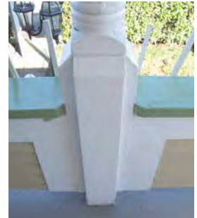
Photos showing top (left) and bottom (right) portion of the typical full lathe turned column and newel post at the front porch. Note the 2x4 addition on above the newel post that is not a character-defining element of Johnston House.
