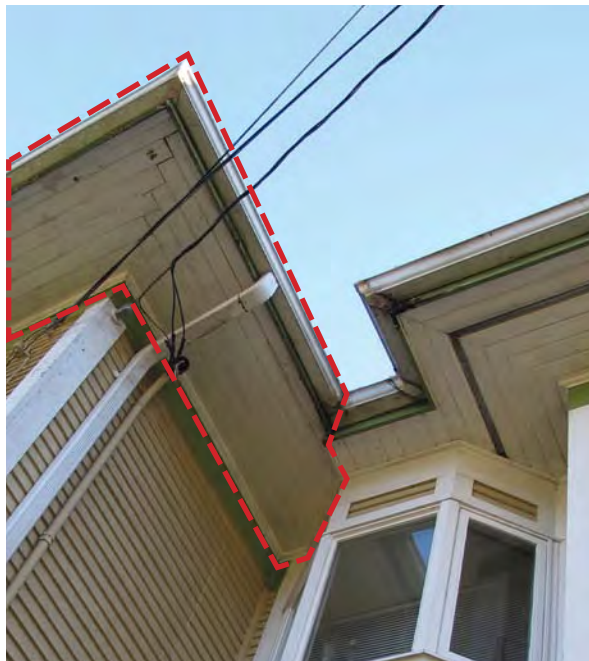
Zig-zag detailing of original wooden board soffits (dashed in red), in comparison with later flush corner detailing of wooden board soffits at the west (left) and east (right) elevations.
