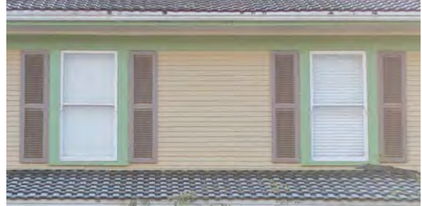
A pair of original double-hung wood-sash windows with wooden horns in symmetrical location above the gable roof of front porch at north elevation.
