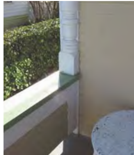
Photos showing top (left) and bottom (right) portion of the engaged lathe turned column at east corner of the front porch.
