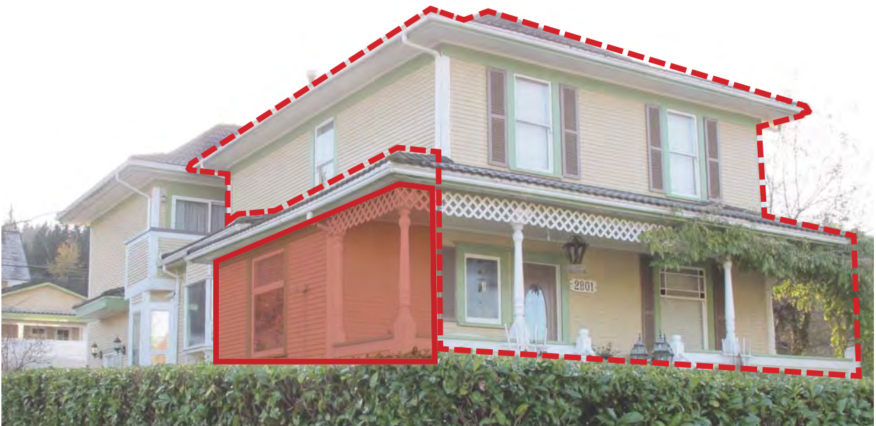
Photo showing partial north (front facade) and east elevations. Note the original Johnston House (dashed in red) and the contemporary side and rear addition (early addition shaded in red).
