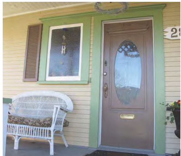
Original door with oval inset glazing and adjacent fixed-pane wood window with frosted glazing.
