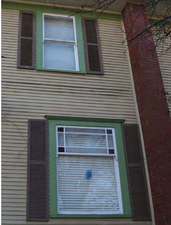
Existing condition of all four original windows at west elevation. Note that all windows on the second floor have similar configuration at west, north, and east elevations. The two ground floor windows at the northwest corner have multi-paned upper sashes and coloured glass.
