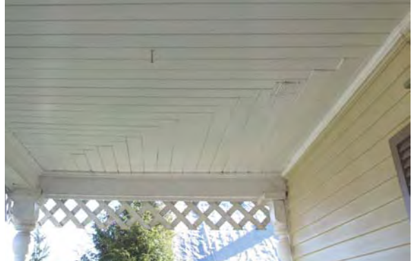
Perpendicular configuration of closed soffit at the east portion of the front verandah.
