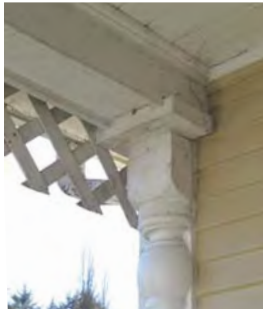
Photos showing top (left) and bottom (right) portion of the engaged lathe turned column at east corner of the front porch.
