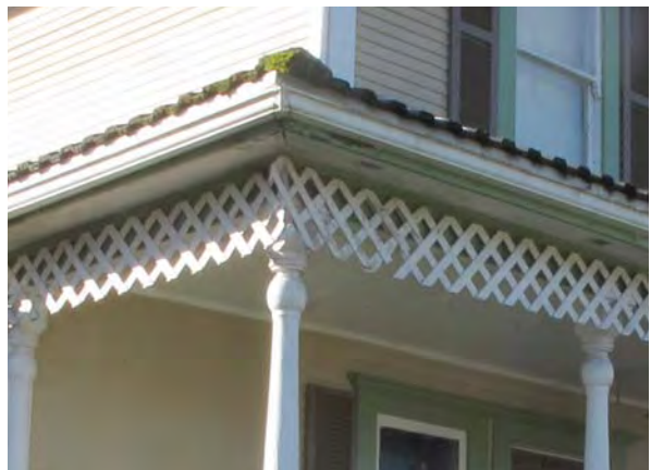
Photo showing original venting along overhang soffit board along the north elevation of the front verandah (missing along the east and west overhang soffits) and decorative wood lattice.
