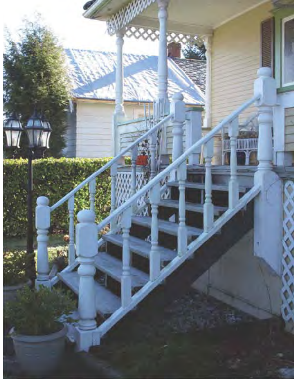
View of existing porch stairs (looking east) showing open balustrade with lathe turned balusters and columns, and newel posts.
