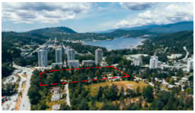
AERIAL VIEW OF SITE LOOKING WEST TOWARDS BUTER BROOK VILLAGE AND BURRARD INLET
