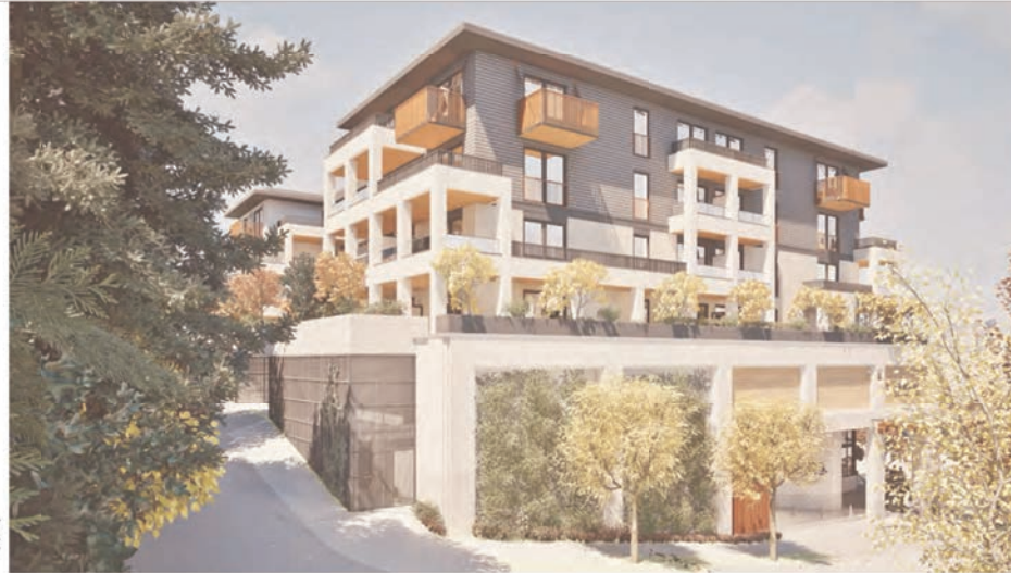
Southeast view from Queens St
