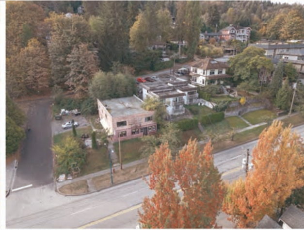
Northeast aerial view
