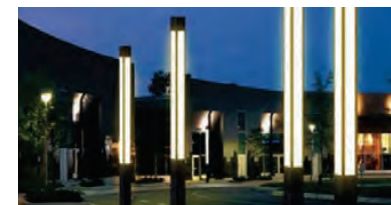
Lighting Integration with Columns
