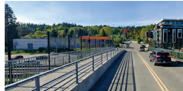
View C. Looking south from Moody St. Source: Google.
