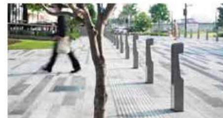
Raised intersection with flush transition to sidewalks, continuous unit paving, bollard, and tactile warning..
