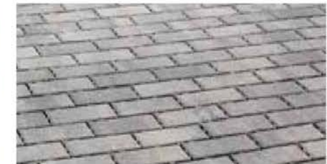
Permeable Pavers at Parking Laybys Belgard Aqualine (110x221.5x80mm), Natural grey or city-approved equivalent
