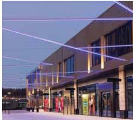
Linear overhead lighting
