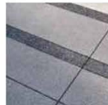
Concrete sidewalk banding
