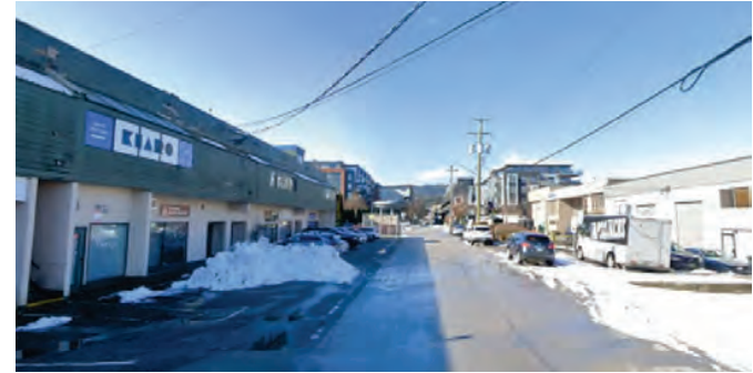
View B. Existing context of Spring St looking east. Source: Google.
