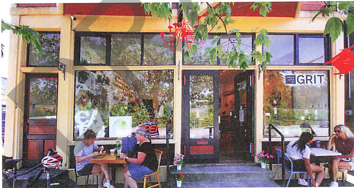
Existing Storefront wood elements: Tapered central posts with chamfered edges flanking main doorway, transom window horizontal banding across entire building facade equally divided into 8 panels, 3 of which are operable; 2 oversized window displays over paneled storefront base; 2 corner end posts and signage banding over transoms framing the main level units.
