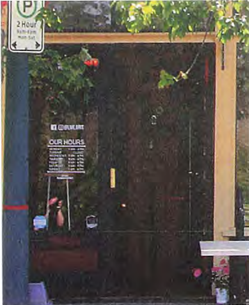
Existing double swing doors of main level commercial space facing Clarke Street. Note original metal mail slot on left paneled combination 3/4 glass and (1) One paneled door.
