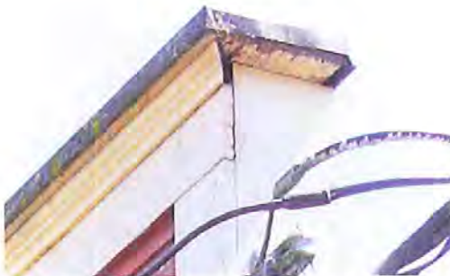
Current state of entablature and metal flashing on left and right sides of the false-front 'Boomtown' facade. Note missing crown mouldings on the returns.
