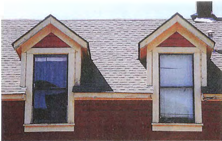
Two sets of extant roof dormers on the East and West elevations of the building with one-over-one, double-hung wood windows appear to have been restored and preserved. Further investigation to determine its condition to be done when possible.
