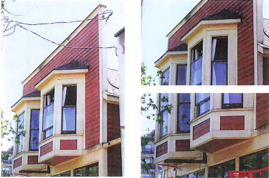
Two extant projecting hexagonal bays above the storefront with three operable double-hung, one-over-one extant wood windows appear to have been restored and preserved.
