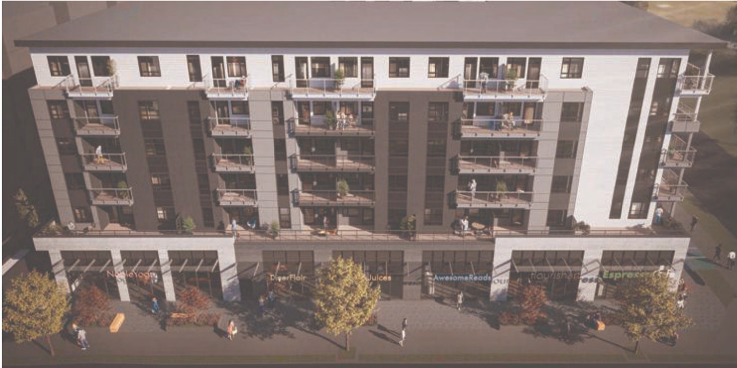
1 St. John's St - Elevation View
