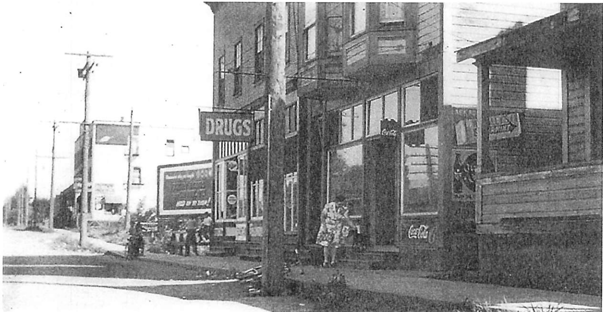
Bottom: South Side of Block 2400 Facing East Circa WW2 (Collection of Valerie Julian). Concrete sidewalk has replaced the original wood decking that existed along Clarke Street. Note the presence of painted signs on all of the commercial buildings advertising their businesses, typical of the era.
