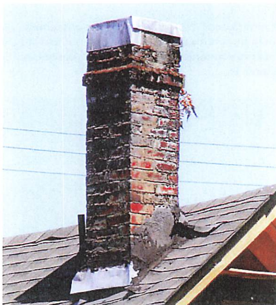
Extant chimney on the southwest side of the roof at the rear of the building.
