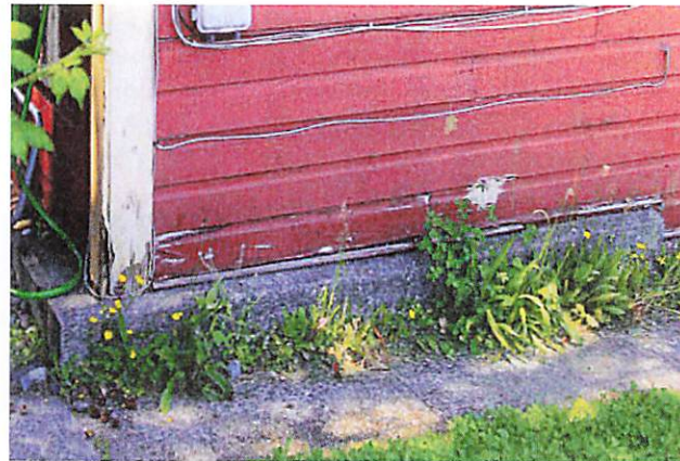
August 2021 East Elevation of building features a stepped poured-in-place concrete foundation following the slope of the site. The intent is to relocate the heritage building to its new location on Spring Street corner Queens Street.
