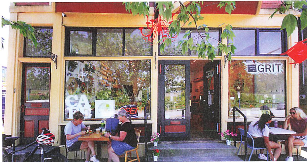
Existing Storefront wood elements: Tapered central posts with chamfered edges flanking main doorway, transom window horizontal banding across entire building facade equally divided into 8 panels, 3 of which are operable; 2 oversized window displays over paneled storefront base; 2 corner end posts and signage banding over transoms framing the main level units.
