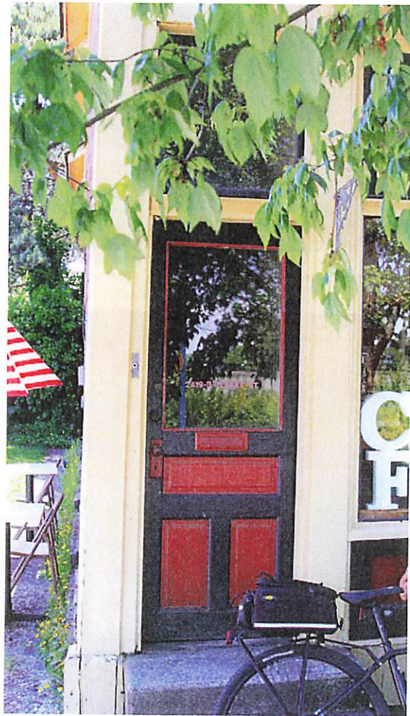
Original door opening on east side of the front elevation provides direct access from Clarke Street. Note metal mail slot, door hardware original to the paneled combination 2/3 glass and (3) Three panelled door.
