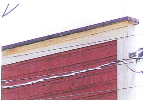
Current state of drop wood sidings on east and north elevations of the building. August 2021. Evidence of cracks, splitting, breaking of wood is visible. Peeling flaking and staining of paint on the facade after decades of exposure to the elements.
