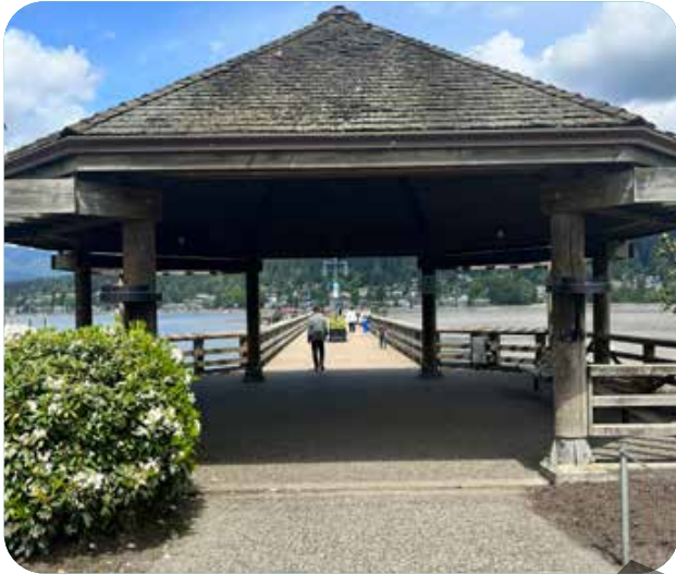
Entrance to the pier
