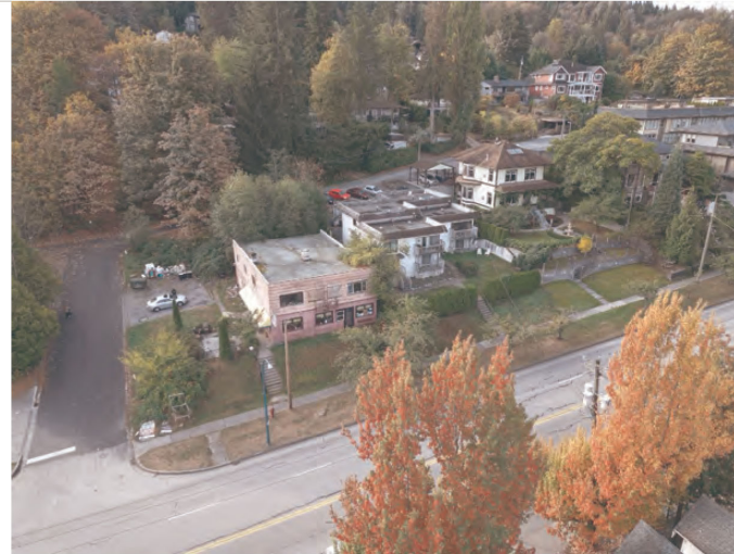
Northeast aerial view
