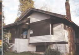
Tremaine Residence 205 Second Ave
