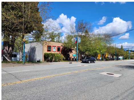
SOUTH - WEST VIEW
