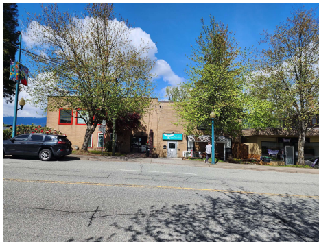
SOUTH / FRONT VIEW
