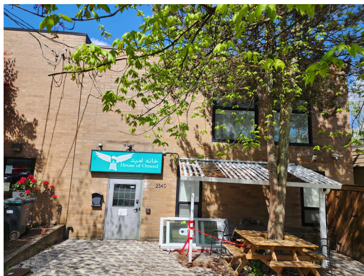
SOUTH / FRONT VIEW
