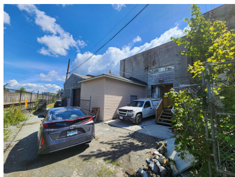
NORTH - WEST VIEW
