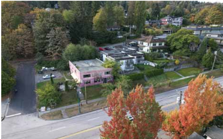
Aerial Photo showing the large grade change and steep slope of Queens and St Andrews as well as the mature trees on the uphill side of St Andrews
