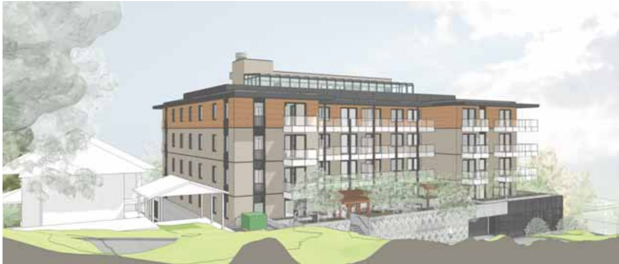
Southwest corner view from the lane
