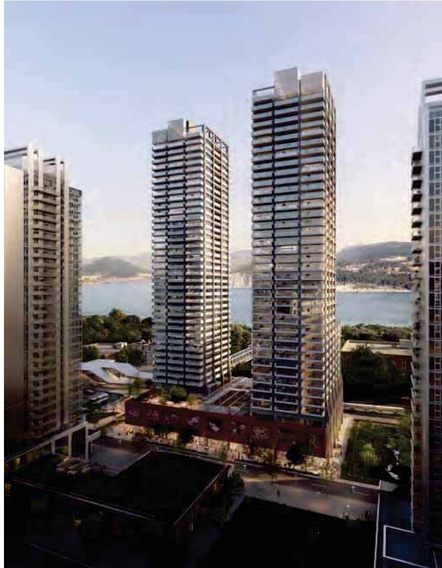
Aerial view of project looking North-West
