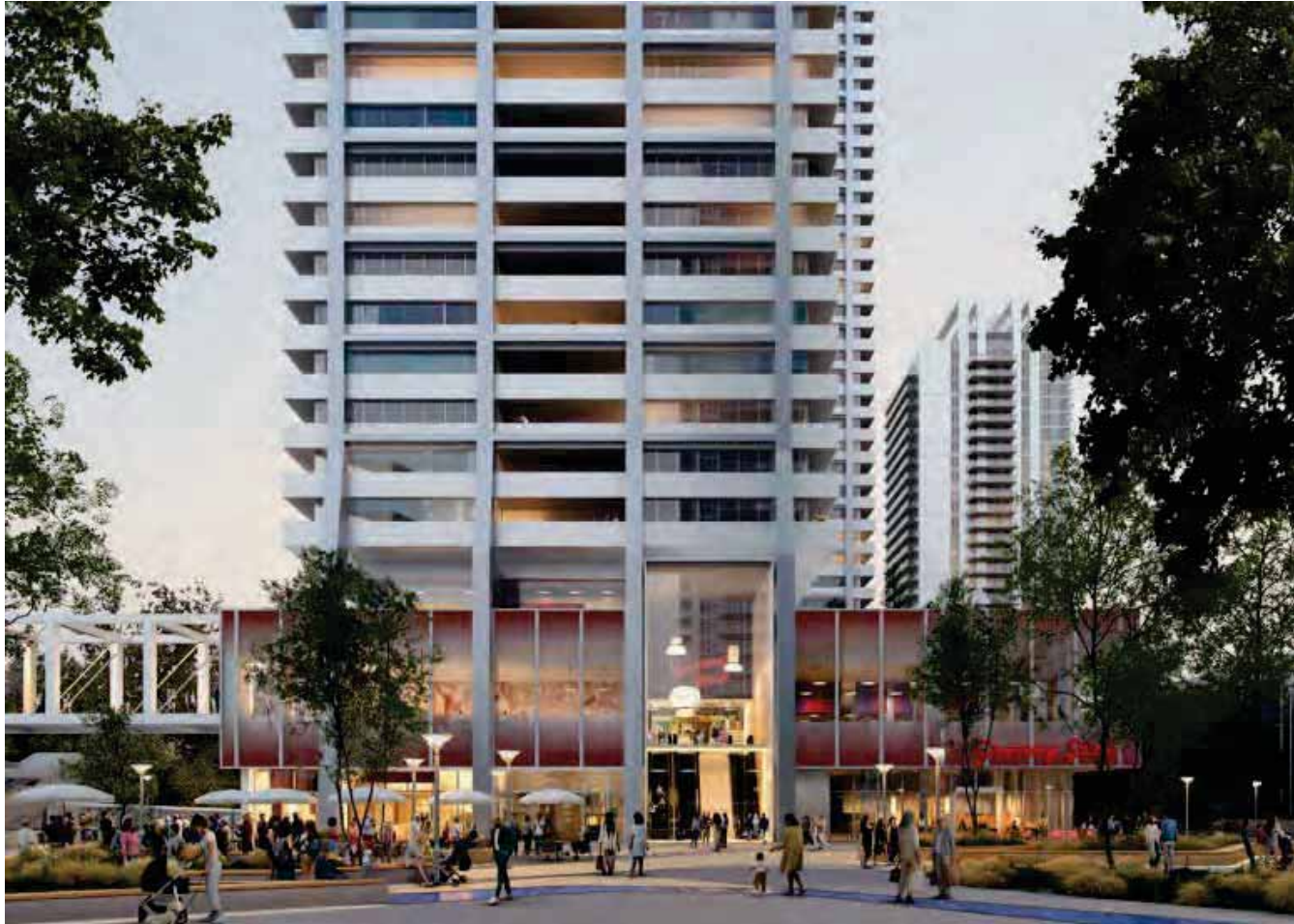
West elevation with community transit plaza in the foreground
