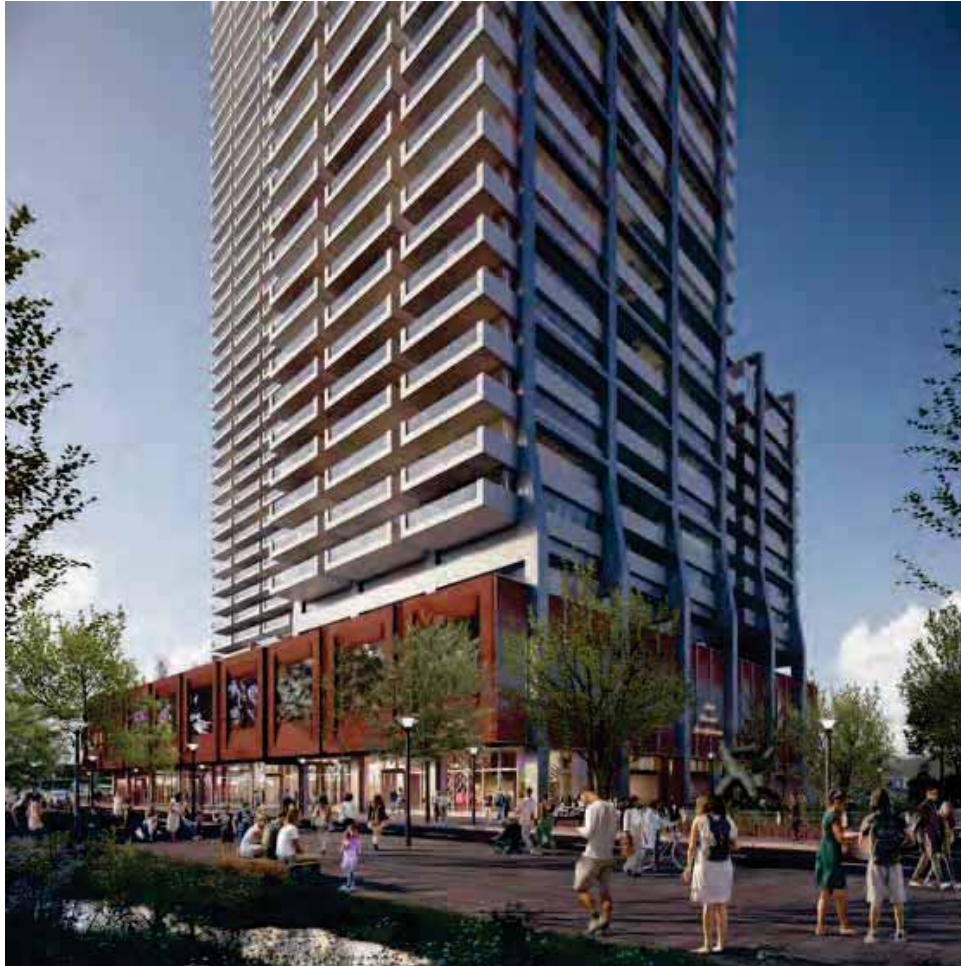
View of South-East corner along Spring Street with ground floor artist space and the Riparian on the right
