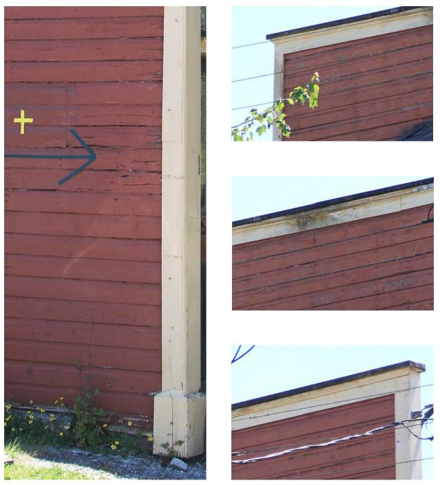
Current state of drop wood sidings on east and north elevations of the building. August 2021. Evidence of cracks, splitting, breaking of wood is visible. Peeling flaking and staining of paint on the facade after decades of exposure to the elements.
