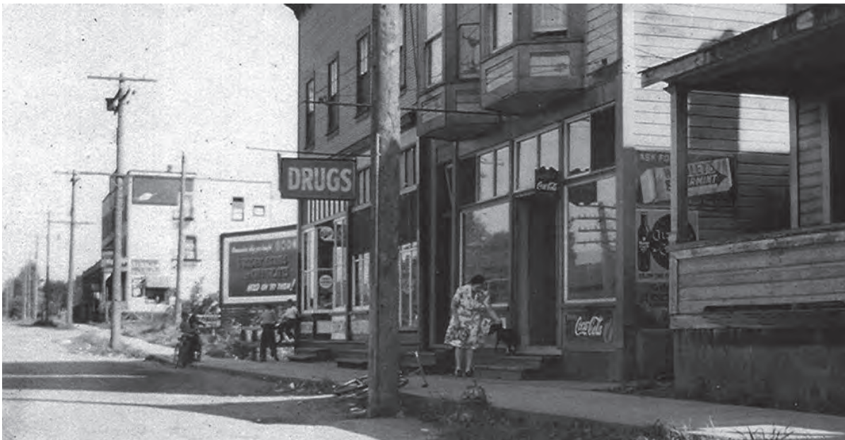
Bottom: South Side of Block 2400 Facing East Circa WW2 (Collection of Valerie Julian). Concrete sidewalk has replaced the original wood decking that existed along Clarke Street. Note the presence of painted signs on all of the commercial buildings advertising their businesses, typical of the era.
