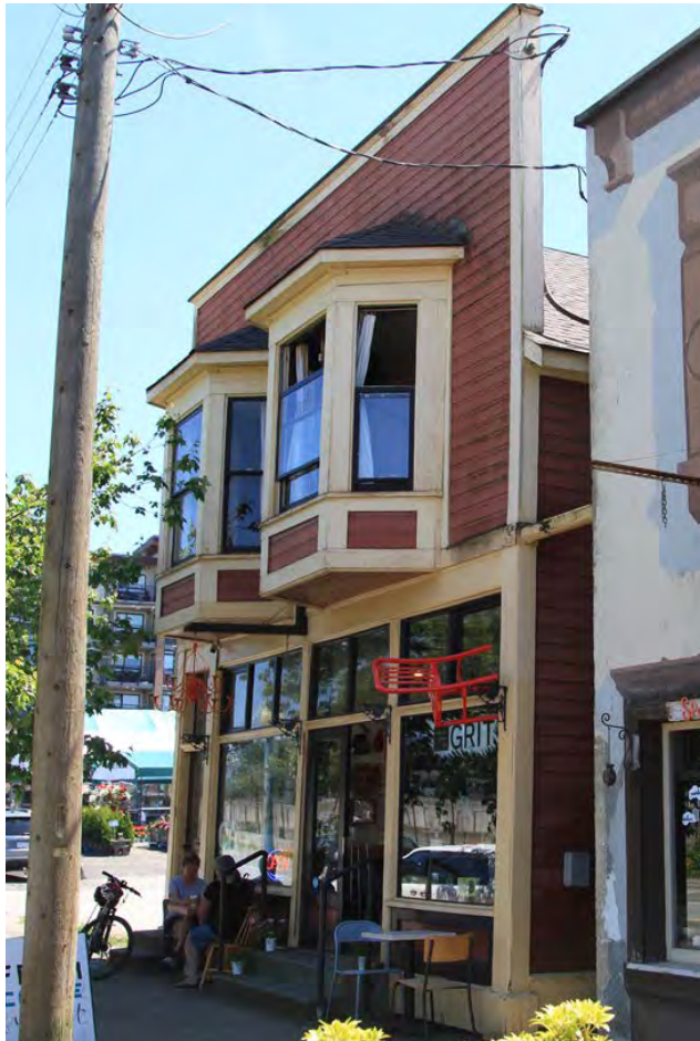
Existing facade of P. Burns & Co. Butcher Shop August 2021.
