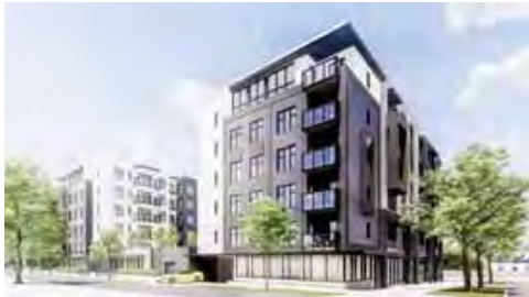
SPRING STREET FRONTAGE @ KYLE STREET
