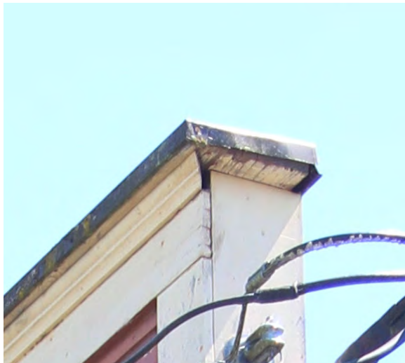
Current state of entablature and metal flashing on left and right sides of the false-front 'Boomtown' facade. Note missing crown mouldings on the returns.
