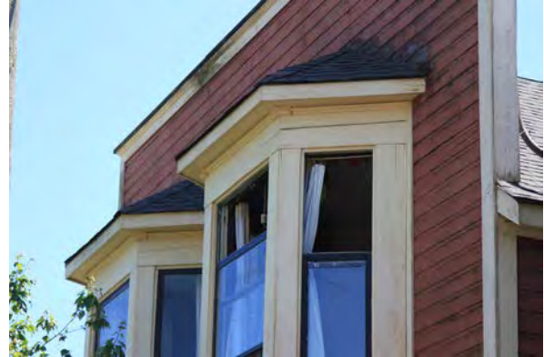
Two sets of extant roof dormers on the East and West elevations of the building with one-over-one, double-hung wood windows appear to have been restored and preserved. Further investigation to determine its condition to be done when possible.
