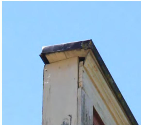
Current state of entablature and metal flashing on left and right sides of the false-front 'Boomtown' facade. Note missing crown mouldings on the returns.
