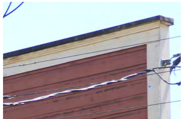
Current state of drop wood sidings on east and north elevations of the building. August 2021. Evidence of cracks, splitting, breaking of wood is visible. Peeling flaking and staining of paint on the facade after decades of exposure to the elements.
