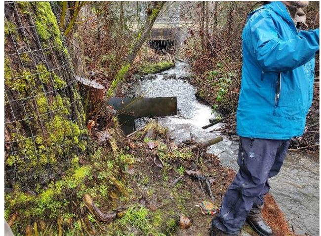
**Photo 6:** View of remaining portions of metal fishway (left bank) taken February 11, 2022
