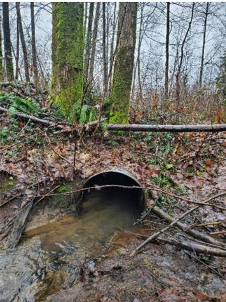
**Photo 9:** Deteriorated culvert conveying the Firehall tributary
