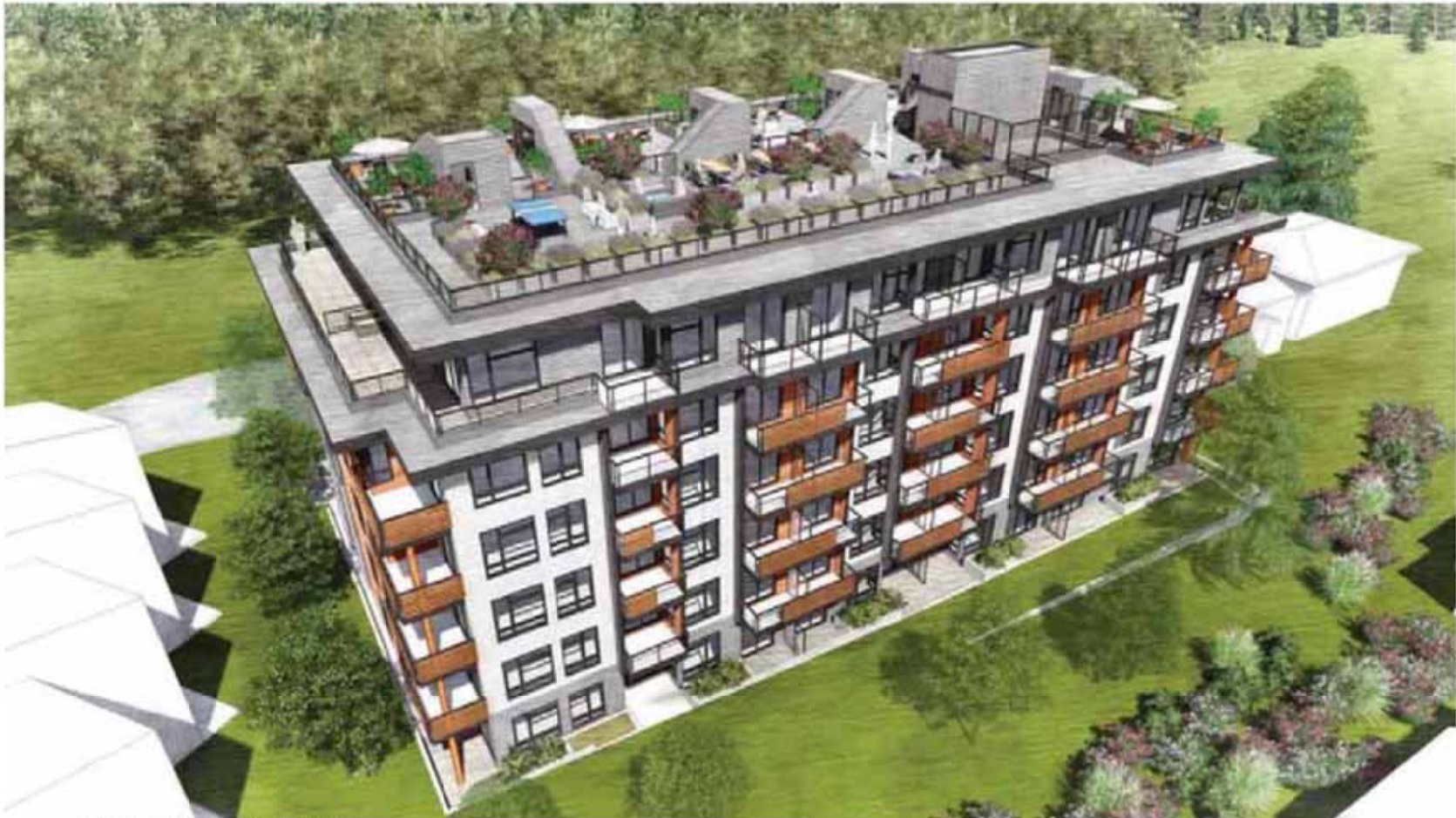
ARIAL VIEW NORTH - ALONG EAST PROPERTY LINE
