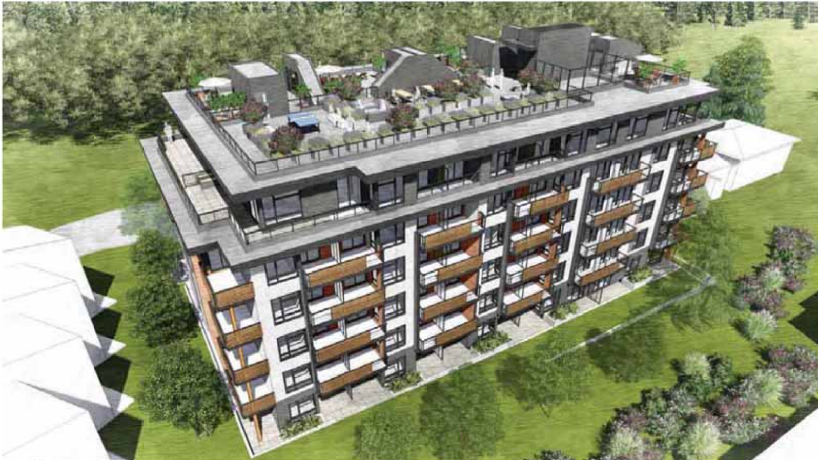
ARIAL VIEW NORTH - ALONG EAST PROPERTY LINE
