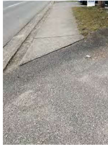
LOCATION 4 St Johns Street (North side) between Hugh Street and Williams Street. Typical sidewalk condition at vehicular entrances to businesses. Almost impossible for wheelchair users to navigate, this is a serious pedestrian issue.
