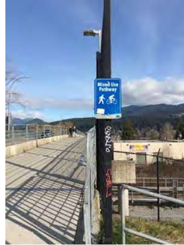
Bridge at Moody Street looking north.
