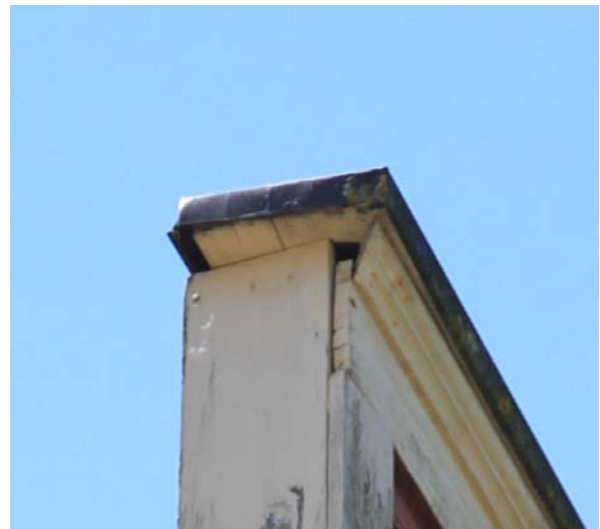
Current state of entablature and metal flashing on left and right sides of the false-front 'Boomtown' facade. Note missing crown mouldings on the returns.
