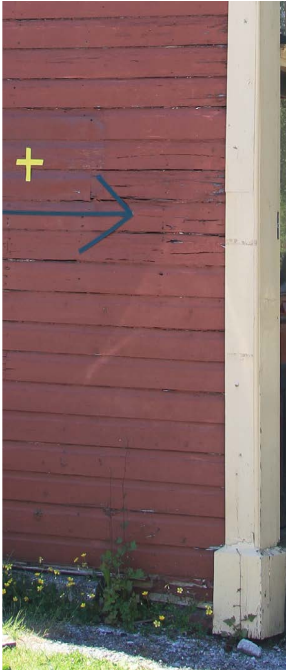
Current state of drop wood sidings on east and north elevations of the building. August 2021. Evidence of cracks, splitting, breaking of wood is visible. Peeling flaking and staining of paint on the facade after decades of exposure to the elements.
