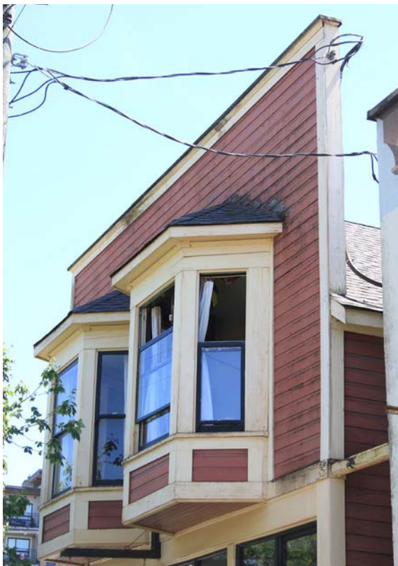
Two extant projecting hexagonal bays above the storefront with three operable double-hung, one-over-one extant wood windows appear to have been restored and preserved.
