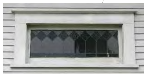
Piano window with leaded and stained glass
