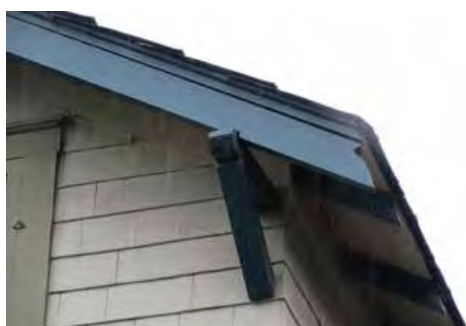
Bargeboard with notched ends
