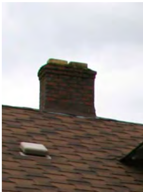
Internal brick chimney with corbelling before removal
