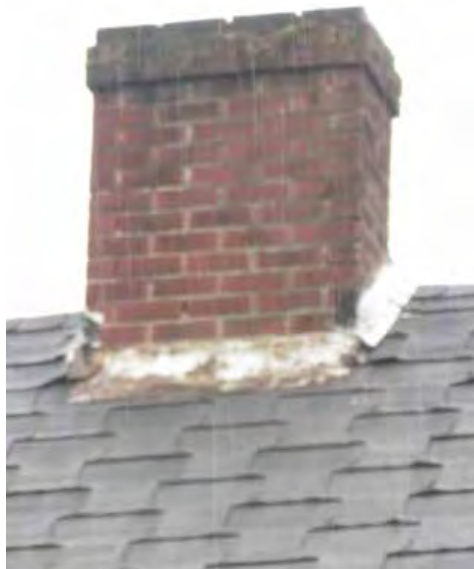
Internal common-red brick chimney
