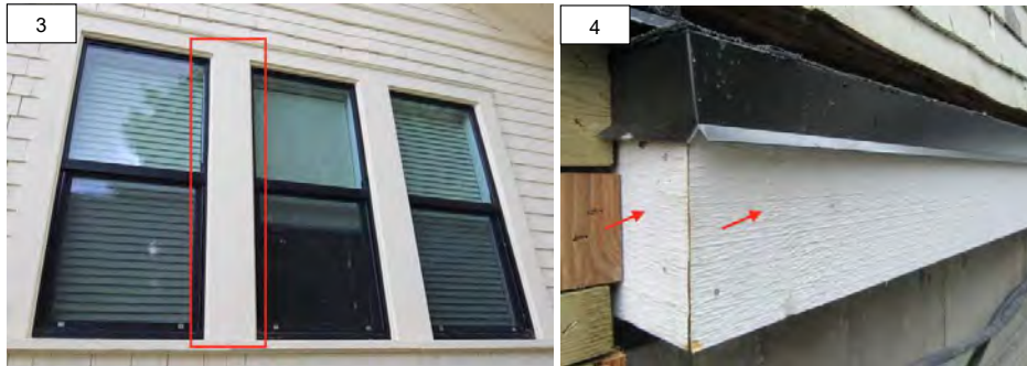
Figure 3 and 4: Detail photos showing textured lumber applications at window casing and watertable.
