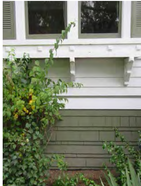
Shingle-clad foundation wall
