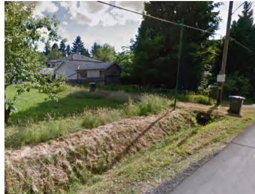
Vintner St. Ditch, Behind 2222 Clarke St. View looking West
