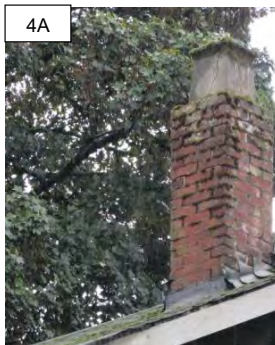
Figure 4A: Internal brick chimney with corbelling before removal.
