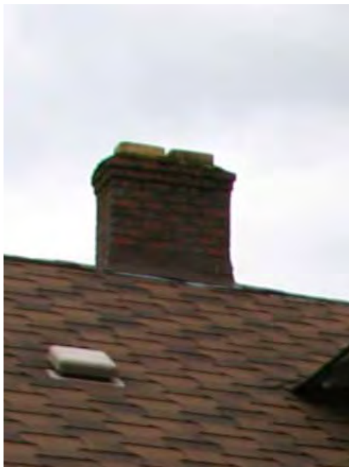
Internal brick chimney with corbelling before removal
