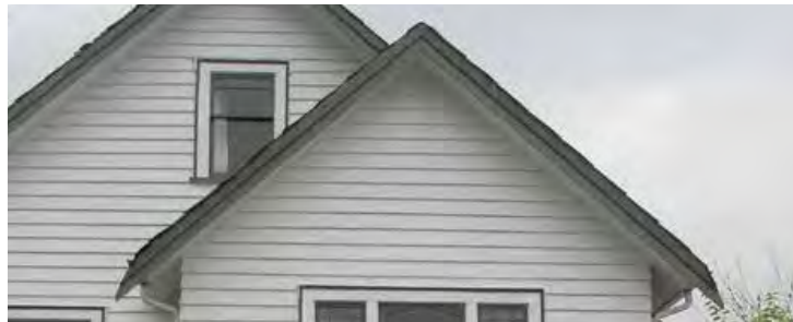
Right: Wooden window trim and bargeboards Bottom: Planter box
