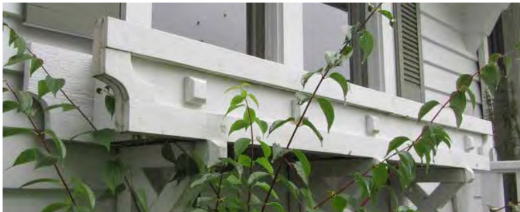
Right: Wooden window trim and bargeboards Bottom: Planter box
