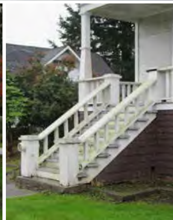
Clockwise from top left: Tongue and groove flooring; Tongue and groove flooring and closed riser; Front porch; Stairs with starting and end newels, and handrails with banisters
