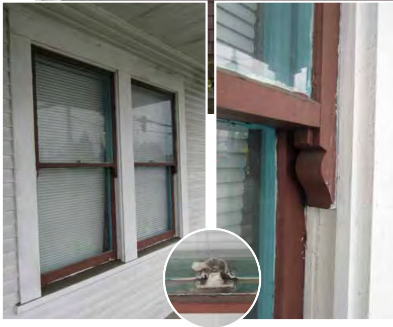
Pair of original one-over-one, double hung wooden sash windows on main floor of front façade with details of sash horn and sash lock
