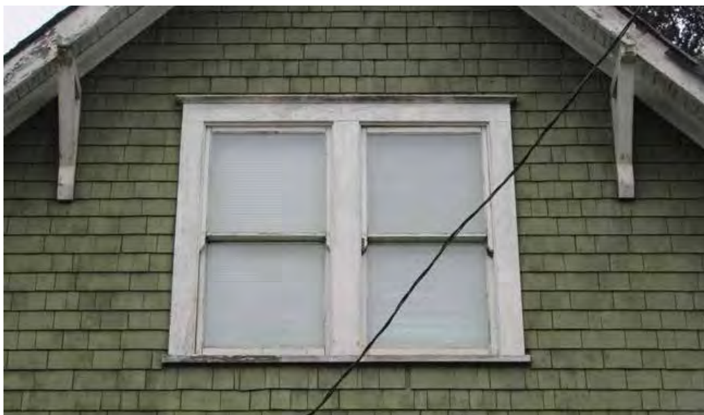
Pair of original one-over-one, double hung wooden sash windows on second storey of front façade
