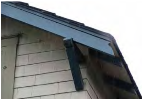
Bargeboard with notched ends
