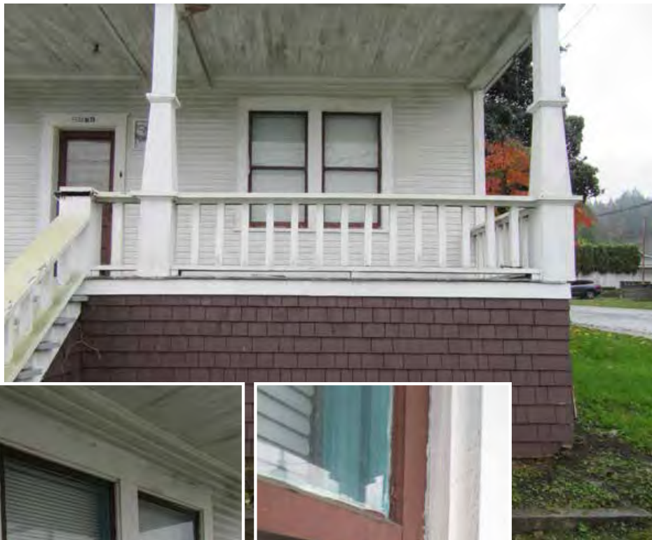
Pair of original one-over-one, double hung wooden sash windows on main floor of front façade with details of sash horn and sash lock
