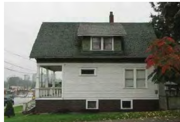
NORTH ELEVATION PHOTO
