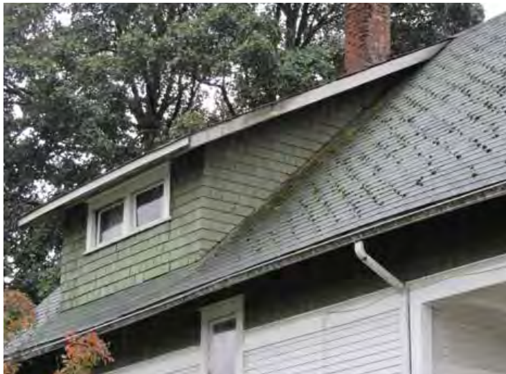
Roof with shed dormer on the east elevation
