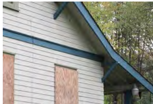
Belt course separating the main and upper floors
