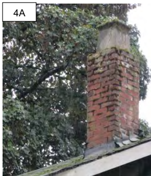
Figure 4A: Internal brick chimney with corbelling before removal.
