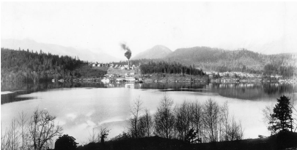
Loco Refinery, 1924, Acc. # 1984.104.001
