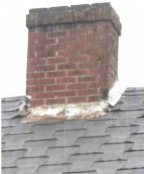
Internal common-red brick chimney
