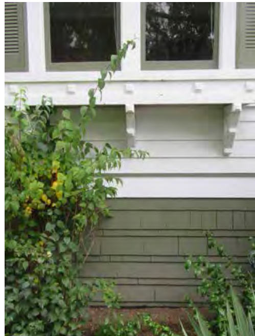
Shingle-clad foundation wall
