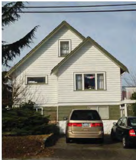
WEST ELEVATION PHOTO
