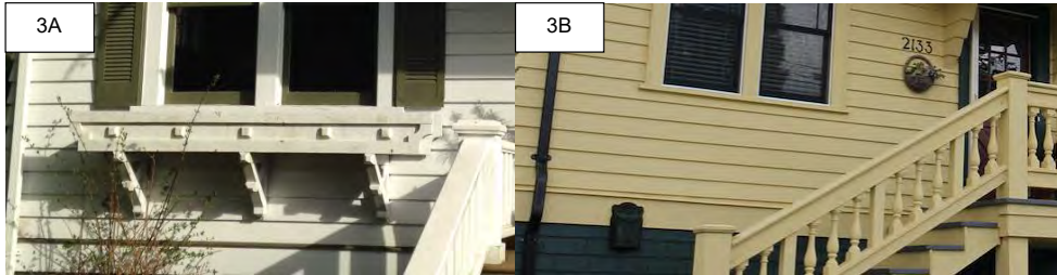
Figure 3A: Front façade wood planter boxes before removal.
