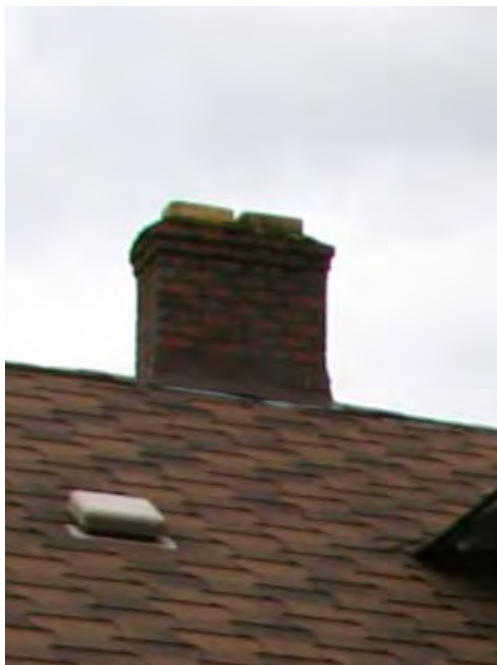
Internal brick chimney with corbelling before removal
