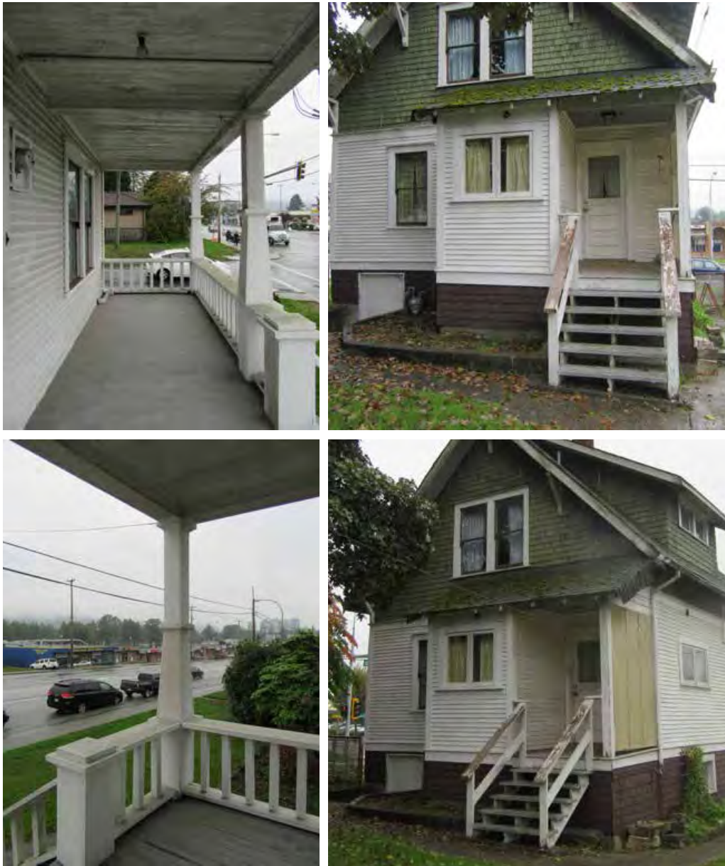
Top Left: Tongue and groove soffit and flooring; Bottom left: Tapered column; Top right and bottom right: Rear porch
