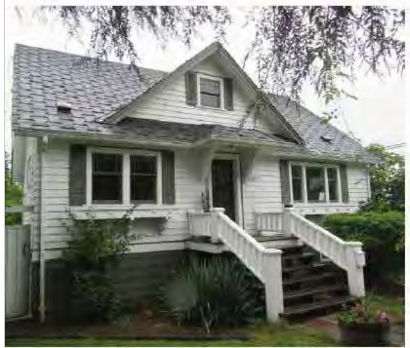
NORTH ELEVATION PHOTO
