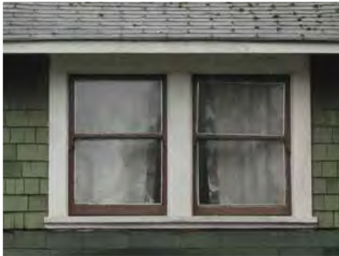
Window assemblies on the west elevation
