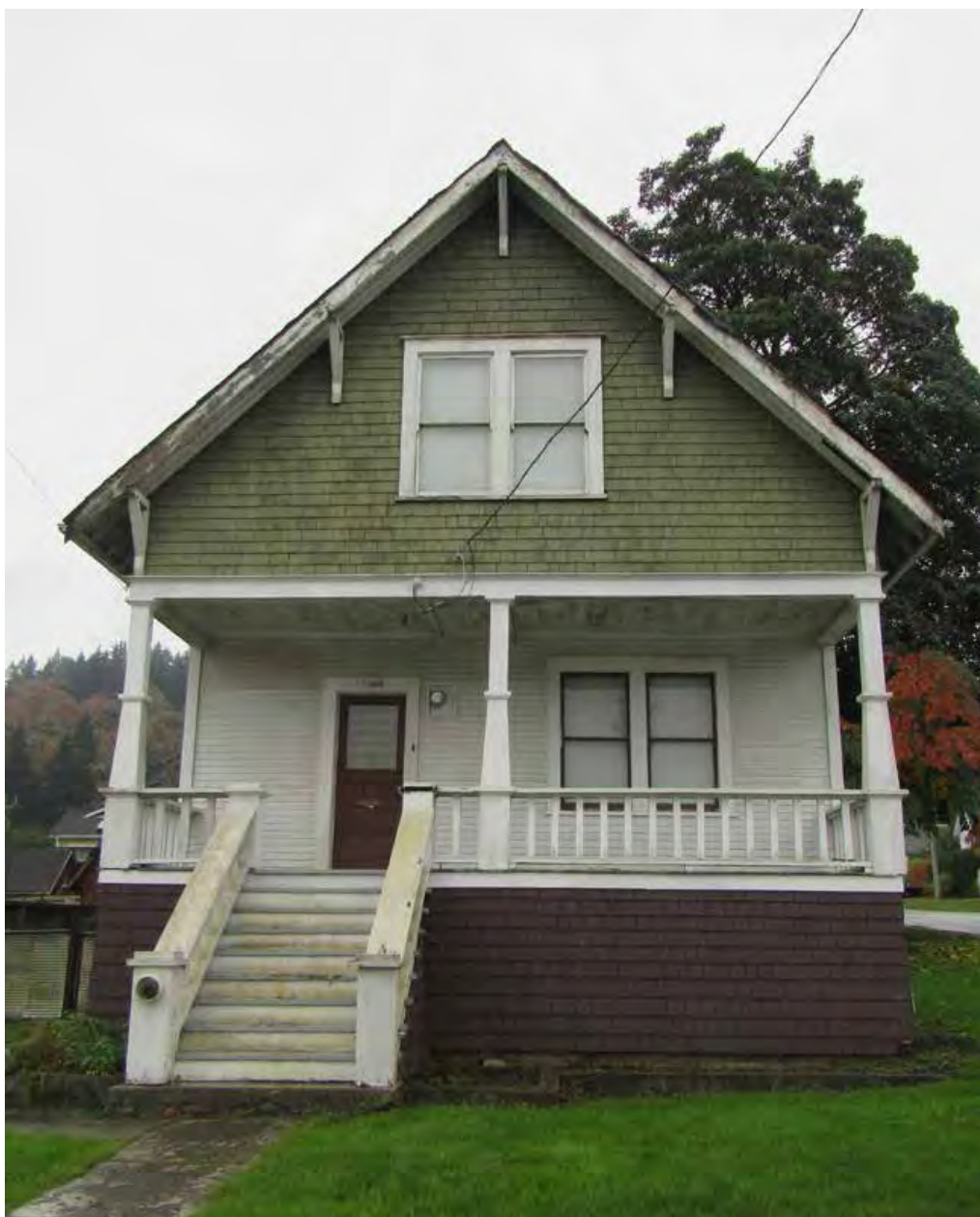
North elevation (St. Johns Street façade), October 2015
