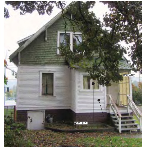
WEST ELEVATION PHOTO
