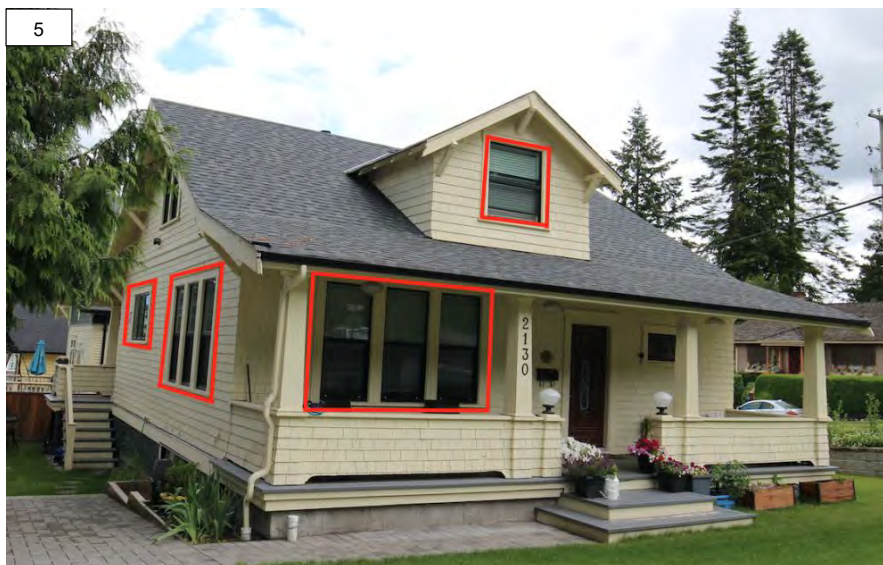
Figure 5: South-west view of Moisio Residence outlining non-wood new and replacement windows.
