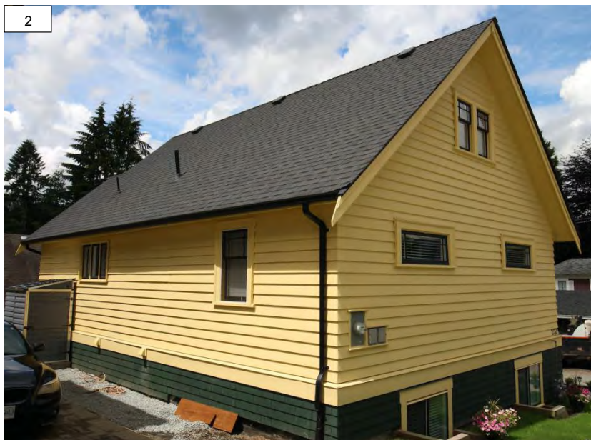
Figure 2: North-west elevation of Sutherland Residence.
