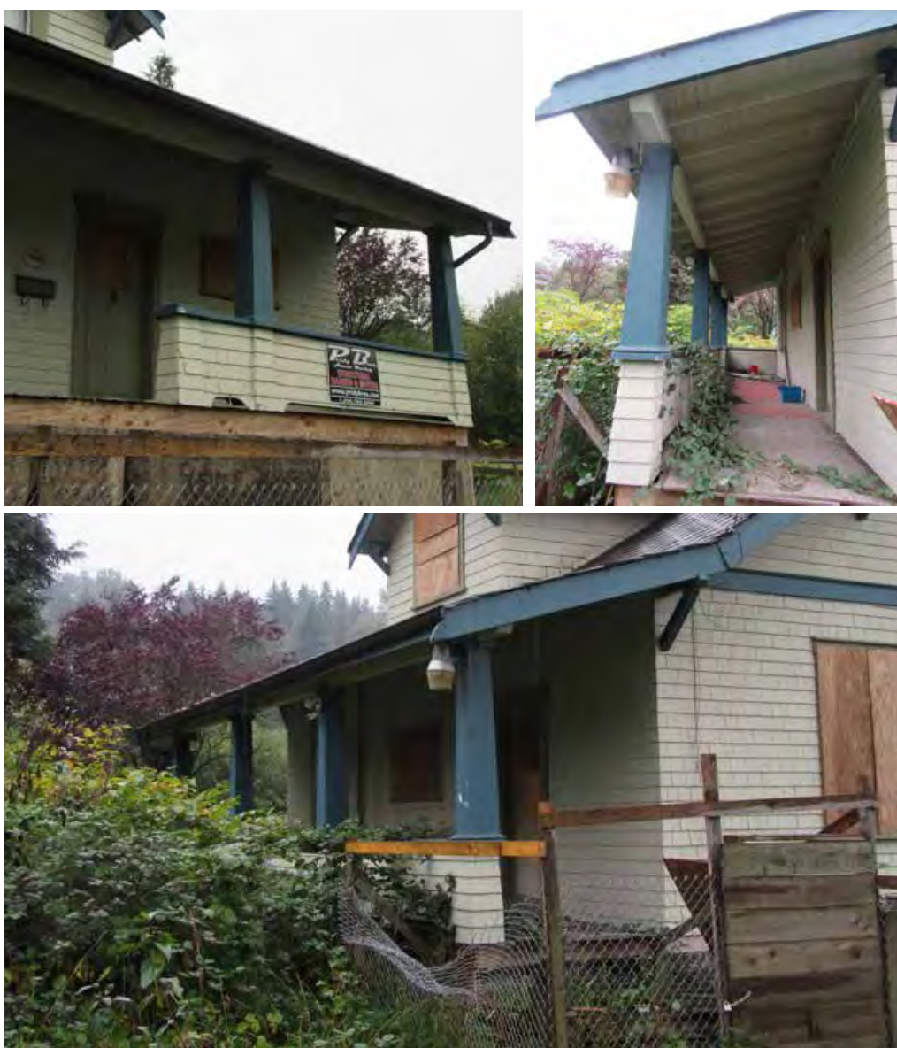
Top Left: Front verandah with tapered columns Top Right: Rear verandah ceiling featuring exposed rafter tails and tongue-and-groove soffits; Bottom: Rear verandah
