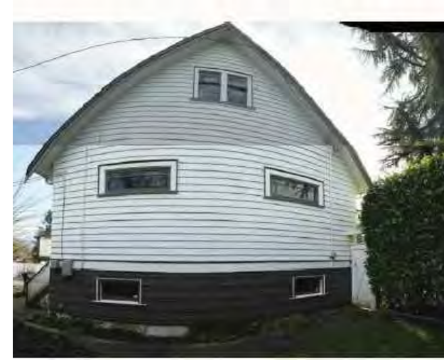
EAST ELEVATION PHOTO
