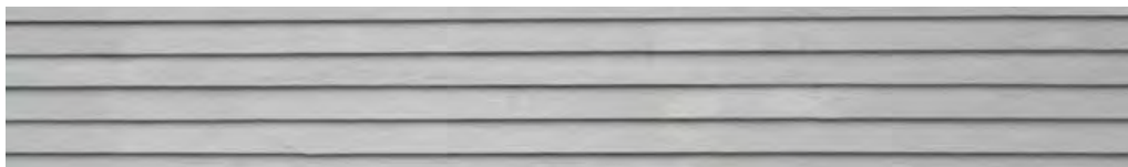
Lap siding, main floor
