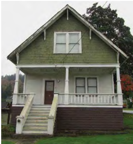
EAST ELEVATION PHOTO
