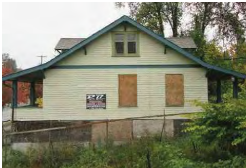
EAST ELEVATION PHOTO
