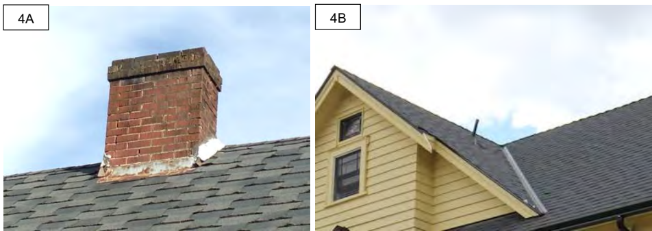
Figure 4A: Internal brick chimney with corbelling before removal.
