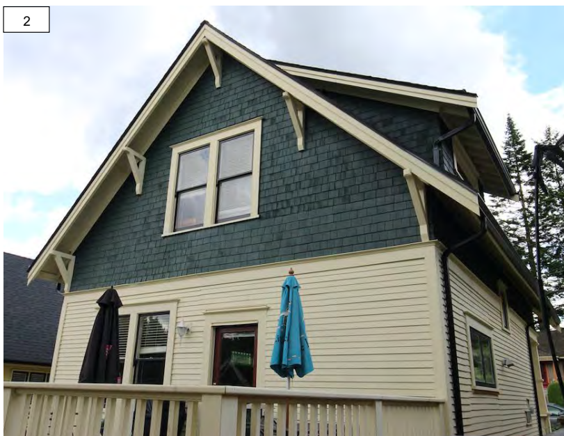
Figure 2: Rear elevation of Siddall Residence.
