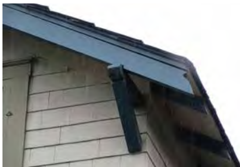
Bargeboard with notched ends
