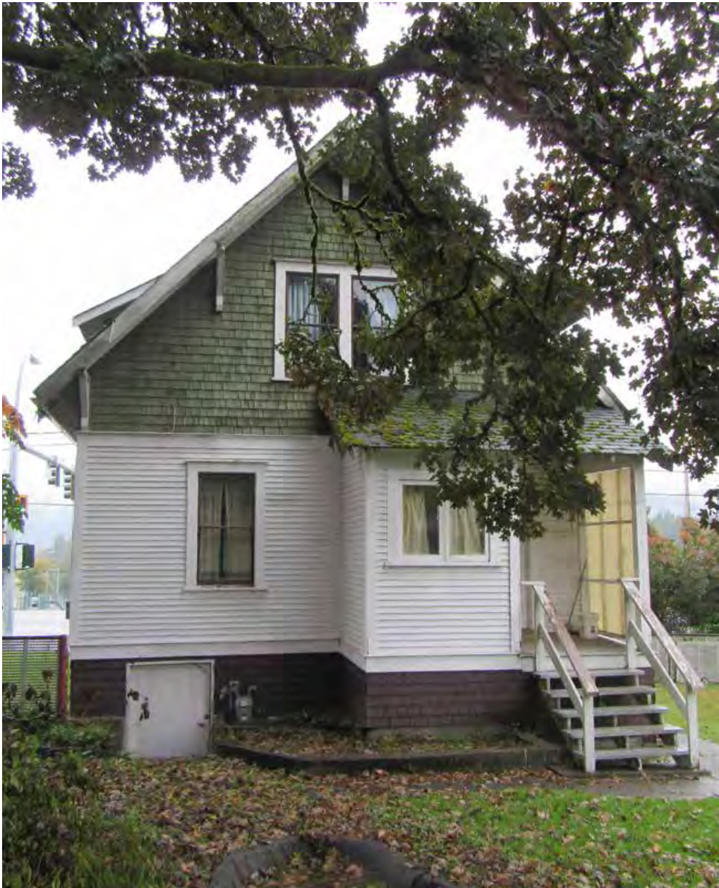
South elevation, October 2015
