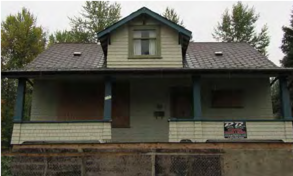
Front verandah with closed and shingled balustrades
