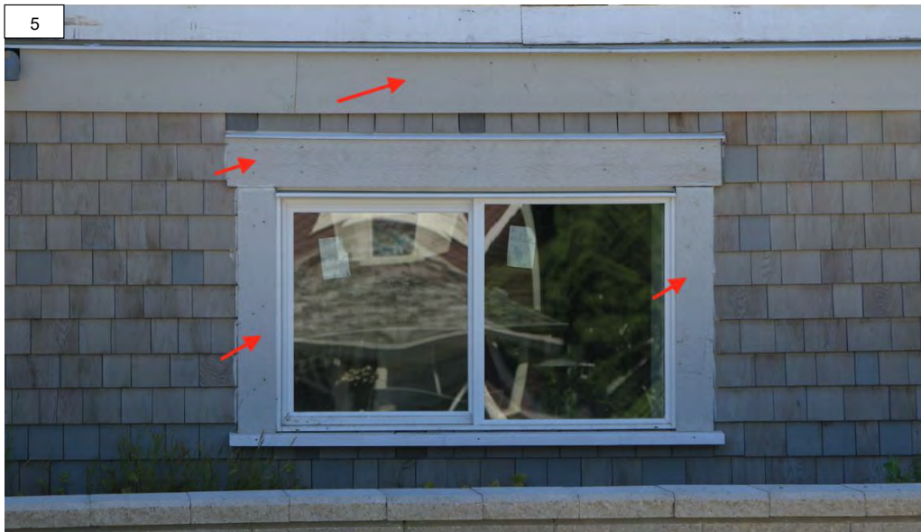
Figure 5: Detail photo showing textured lumber applications at window casing and watertable prior to painting.
