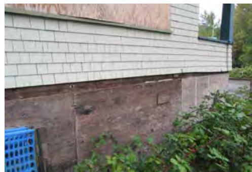
Cedar shingles on main floor and plywood at basement level
