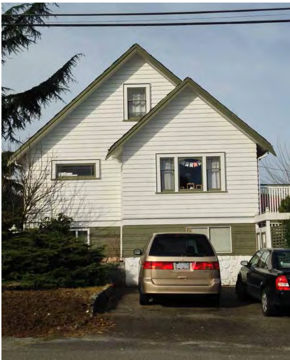
East elevation, March 2016
