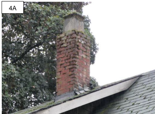
Figure 4A: Internal brick chimney with corbelling before removal.
