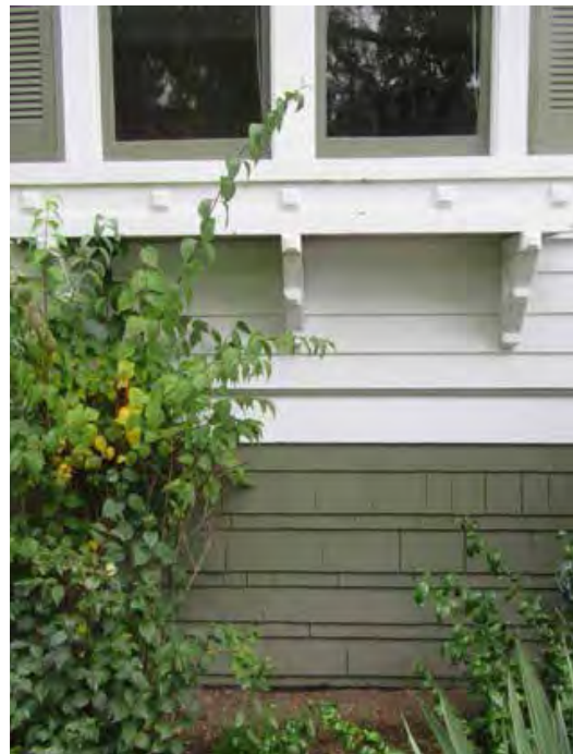
Shingle-clad foundation wall
