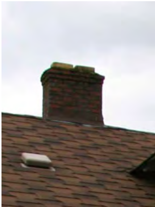
Internal brick chimney with corbelling before removal
