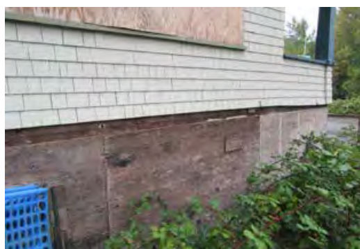
Cedar shingles on main floor and plywood at basement level
