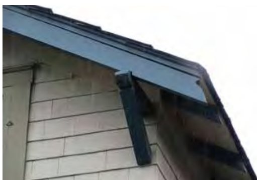
Bargeboard with notched ends
