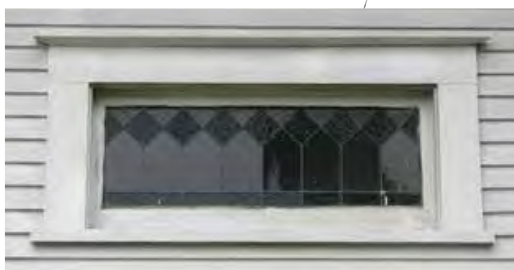
Piano window with leaded and stained glass
