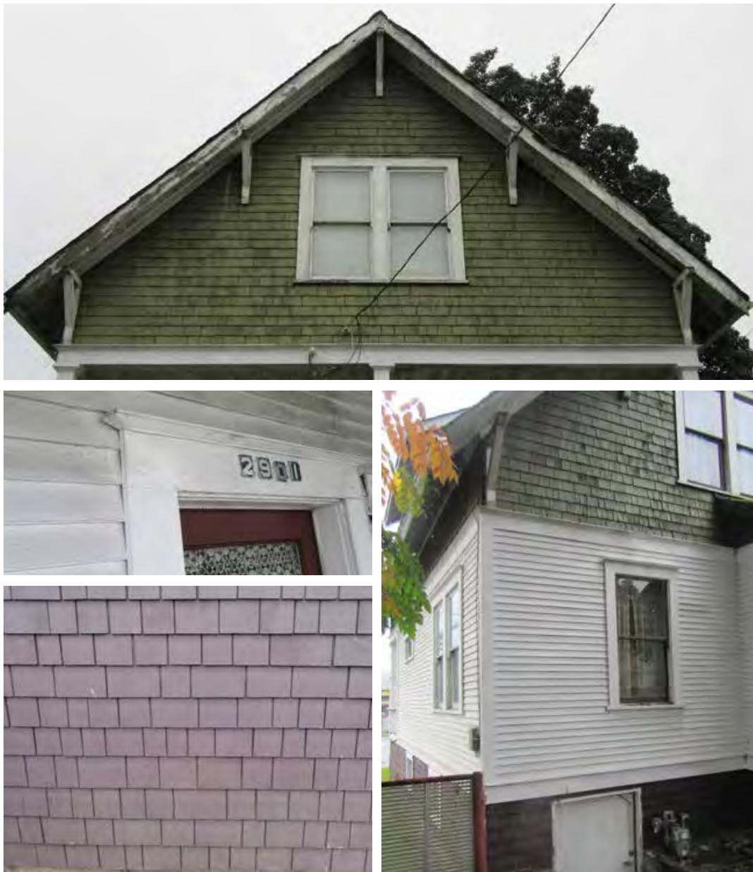
Clockwise from Top: Shingle siding at second floor; Lap siding, belt course, watertable and cornerboard; Shingle siding at basement; Door trim
