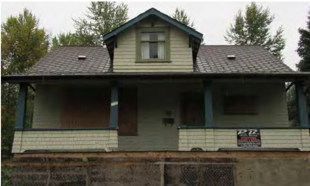
Front verandah with closed and shingled balustrades
