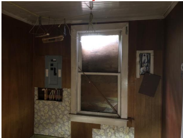
Figure 10: North Side (Front) Porch – corresponding double-hung window.
