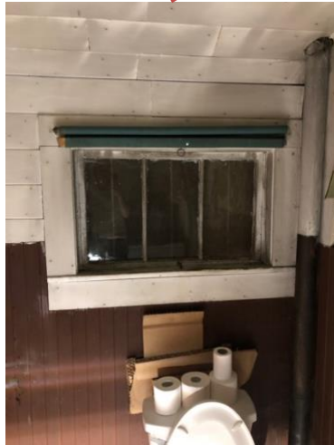
Figure 8: East Side – corresponding windows: all are awning operation. This is the only section of the house with a gutter remaining.
