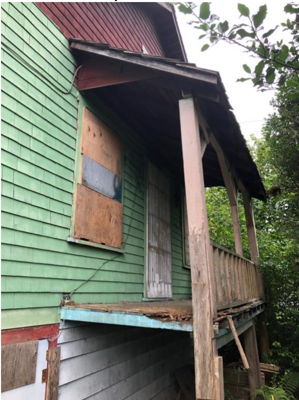
Figure 11: Full view of Front Porch along North Side, illustrating the deteriorated condition of the porch floor and sub-structure.
