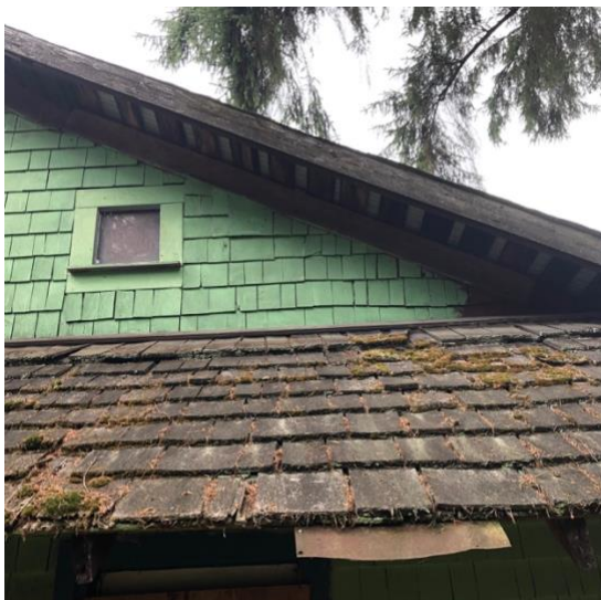
Figure 13: Condition of Soffit and Roof Structure, South Side Overhang
