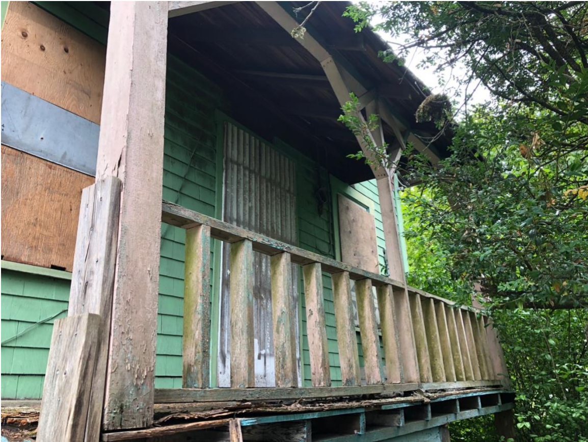
Figure 11: Full view of Front Porch along North Side, illustrating the deteriorated condition of the porch floor and sub-structure.
