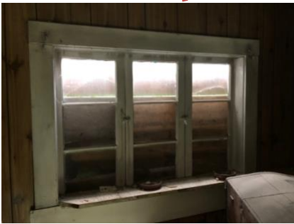
Figure 7: South Side – corresponding windows: (left to right) casement with fixed centre, casement/fixed, fixed.
