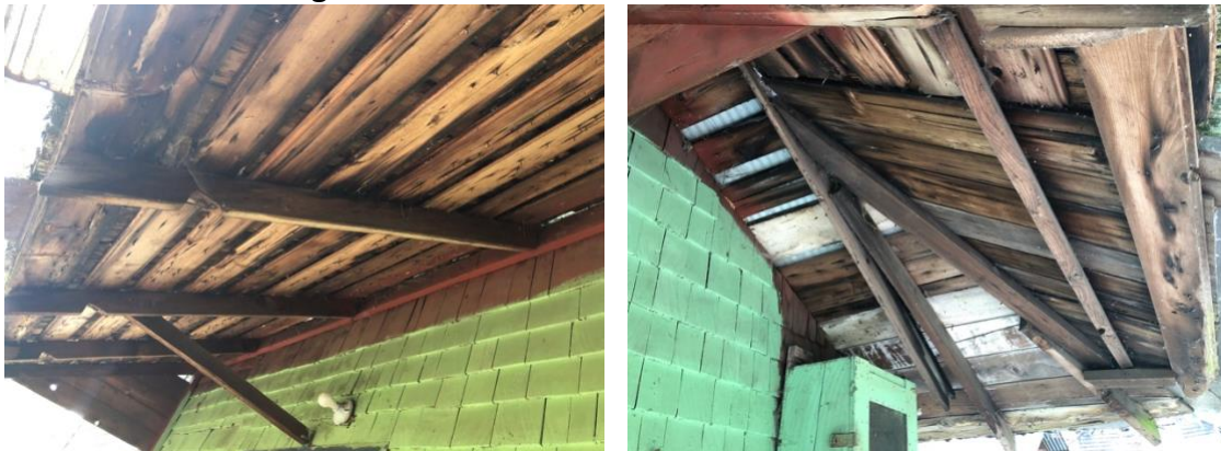
Figure 13: Condition of Soffit and Roof Structure, South Side Overhang
