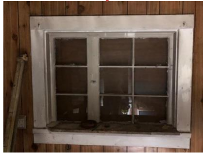
Figure 7: South Side – corresponding windows: (left to right) casement with fixed centre, casement/fixed, fixed.
