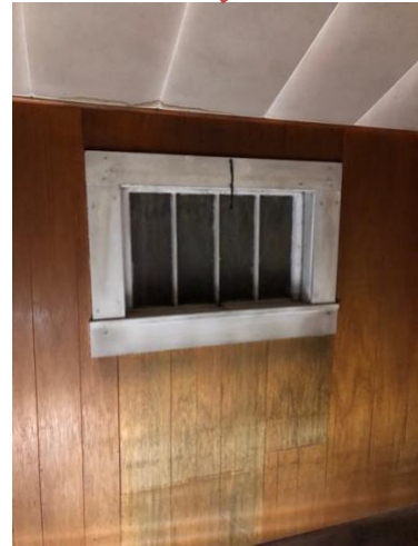
Figure 8: East Side – corresponding windows: all are awning operation. This is the only section of the house with a gutter remaining.
