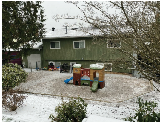
REAR VIEW 1 (SOUTH)
