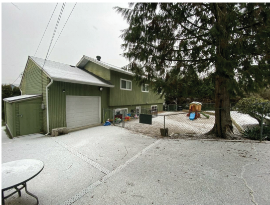
REAR VIEW 2 (SOUTH WEST)
