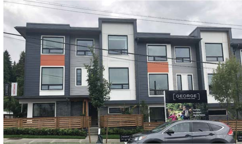
ST. GEORGE FACING SOUTH
