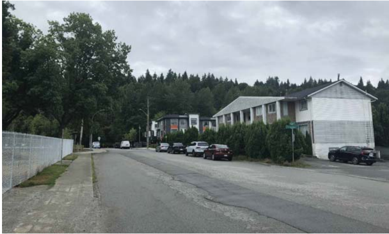
BULLER AND ST. ANDREWS LOOKING SOUTHWEST
