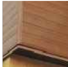
METAL CLADDING - WOODGRAIN
